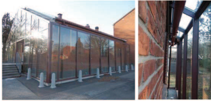
Fig. 1. Added glass façade on the brick building with south façade to the left and east façade to the right.
