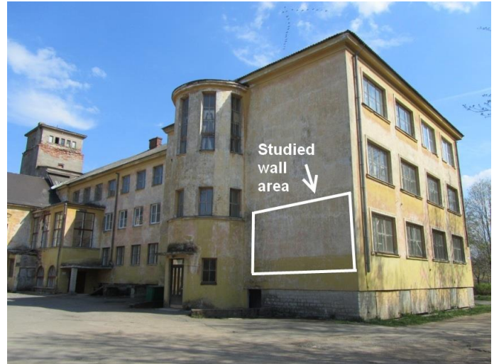
Figure 1. View of the studied school building.
