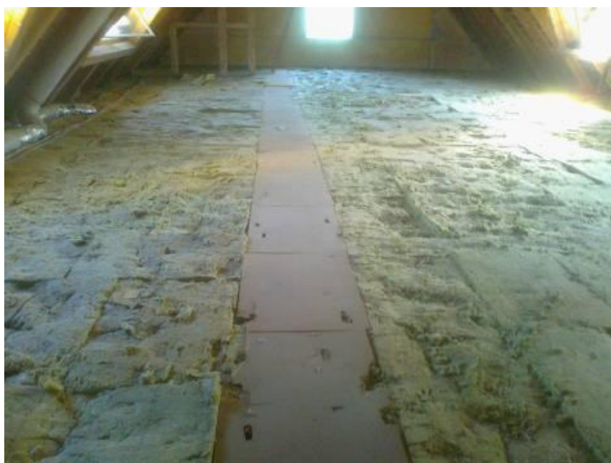
Photo 21. Unheated attic with existing insulation on top of the floor. Thermal insulation was improved by injecting the hollow floor with loose-fill insulation.
