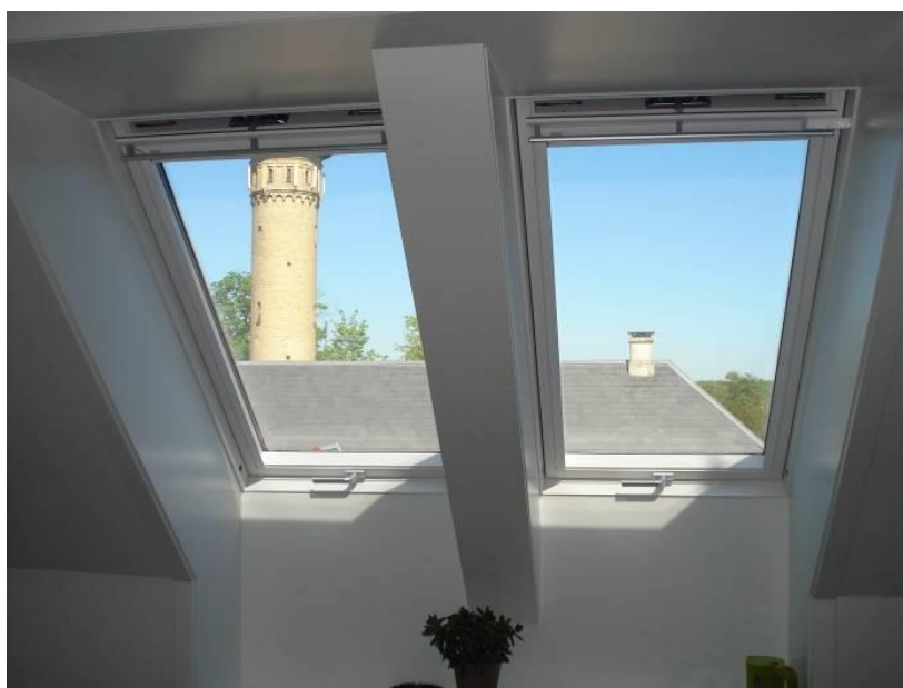
Photo 9. VELUX roof windows placed 2 by 2 to the north.
