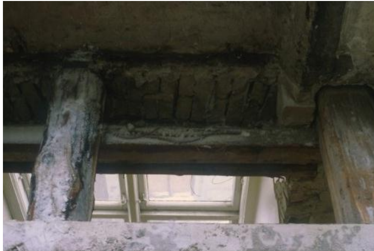
Photo 6. Load-bearing timber beams and timber wall plate at window recess in typical Danish multi-storey building with solid brick walls.
