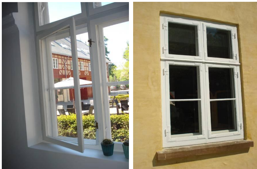
Photo 8. Storm windows with new energy-efficient glass and sealing strips (left). Typical wooden “Dannebrogs” window with characteristic hinges and angle iron (right)
