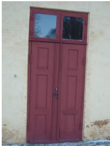
Photo 11. Two doors were repaired and storm windows installed above.
