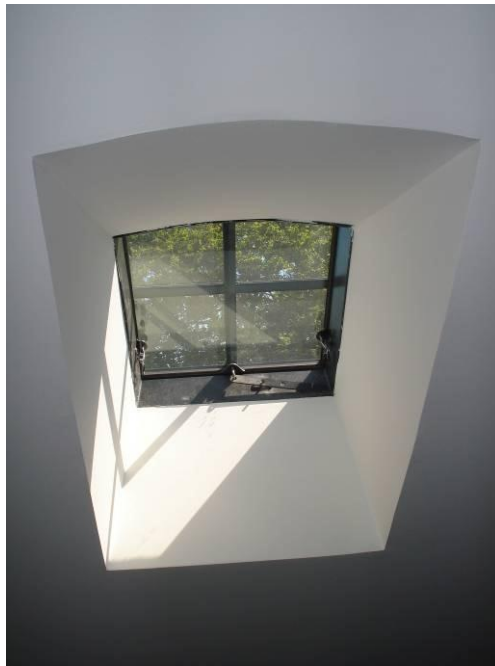
Photo 10. Cast iron roof window (GH Holbæk Jernstøberi) after the refurbishment
