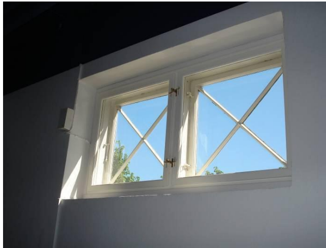
Photo 15. Small sized window with striking glazing bars. The thermal performance was improved by installing storm windows with energy-efficient glazing.
