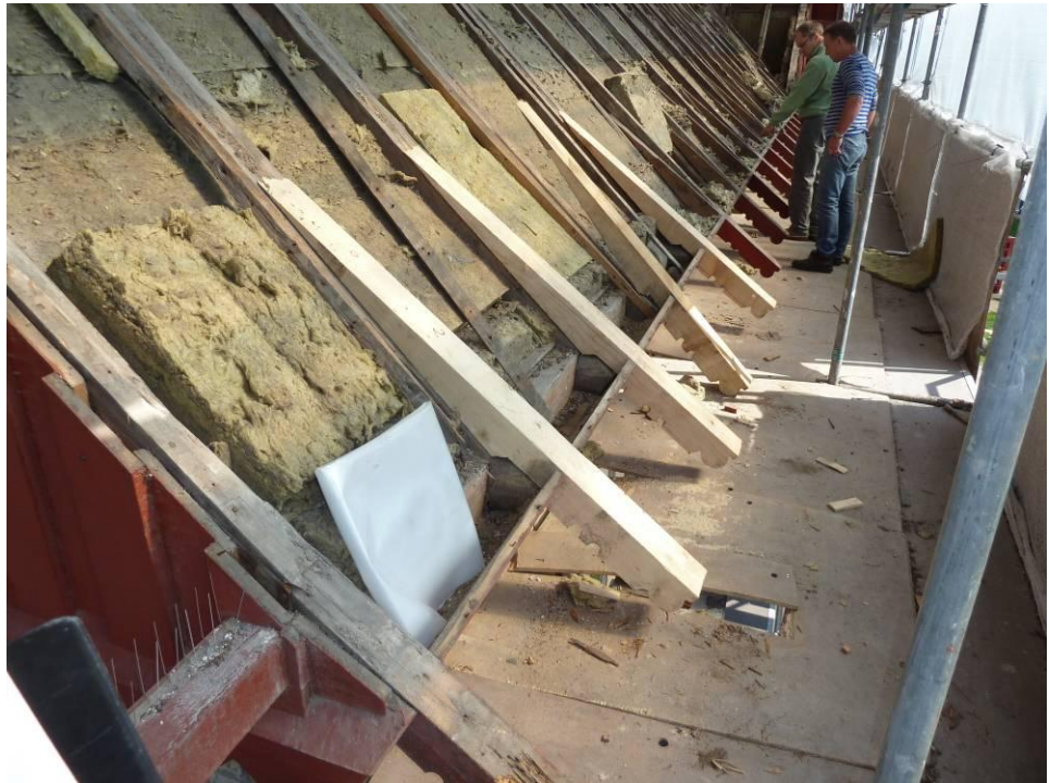
Photo 13. Eave without roof covering showing insulation and specially fitted eaves boards
