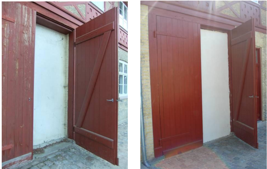
Photo 18. Covered door before and after repair and improved thermal insulation.
