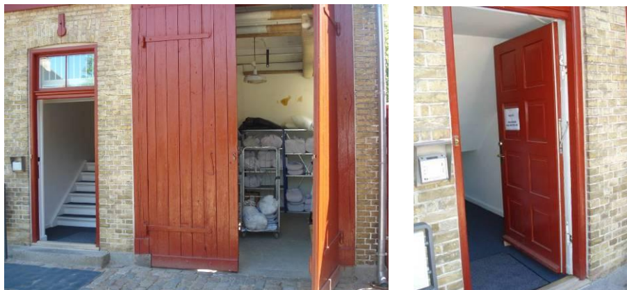
Photo 16. The door leaf was replaced and storm windows installed above the door.
