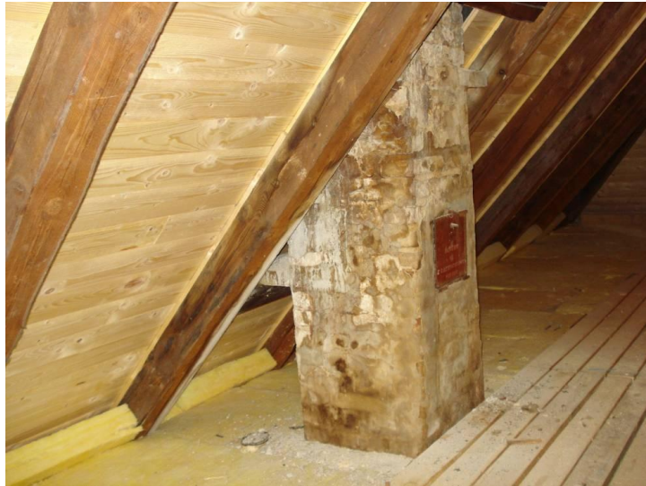
Photo 19. A view from the unheated loft showing insulation, rafters, under-roof, chimney and boardwalk.
