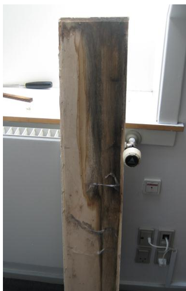
Photo 7. Wooden beam from the old roof construction attacked by mould.
