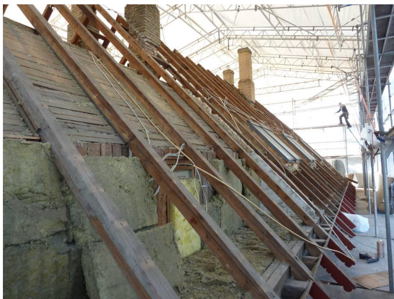
Photo 20. Roof before improved thermal insulation.
