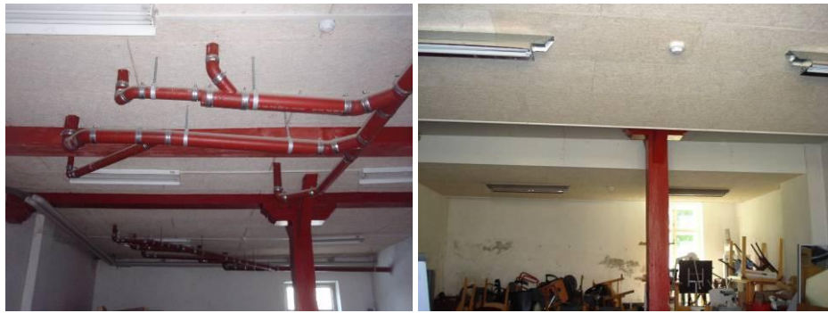
Photo 12. Ceiling in depot/garage before and after insulation. Pipes were moved to the area with wooden columns and beams.
