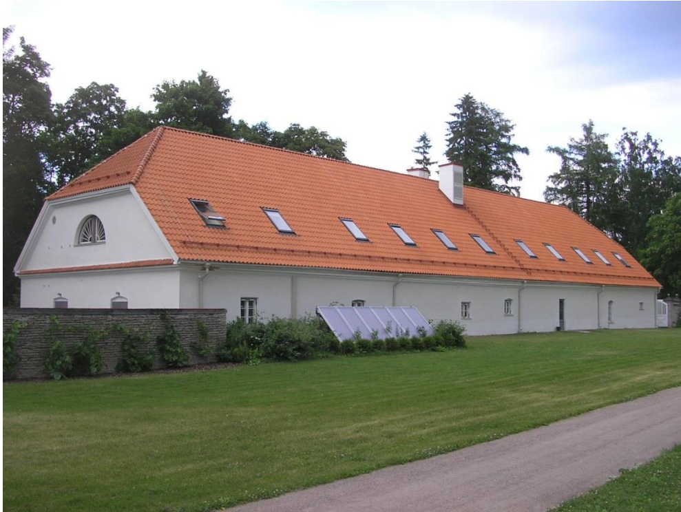
Figure 3 Vihula mõisa conference centre. Part of the hotel DHW is prepared using solar collectors. Building heat supply is ground-source heat pump. Source: Restor
