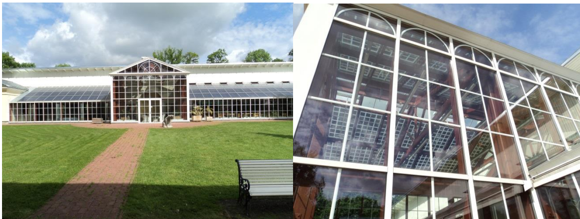
Figure 4 Mäetaguse mõisa conservatory-bathhouse. Glass-roof is covered with solar panels that produce electricity and let the light in, while protecting the space from overheating. Source: Restor
