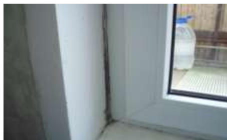
Fig.3.18. The growth of mould results as poor indoor climate
