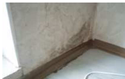
Fig.3.18. The growth of mould results as poor indoor climate
