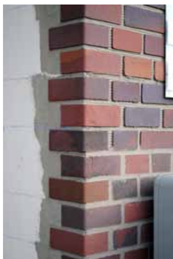
Just a brick illusion: Insulation of the outer wall, Hamburg, Germany
