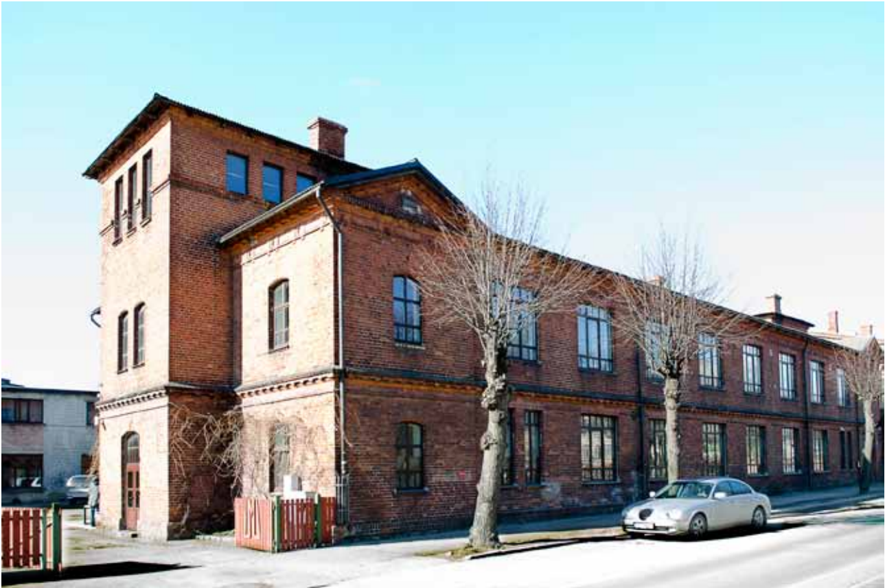
Brick building in Alejas street, Liepaja, Latvia
