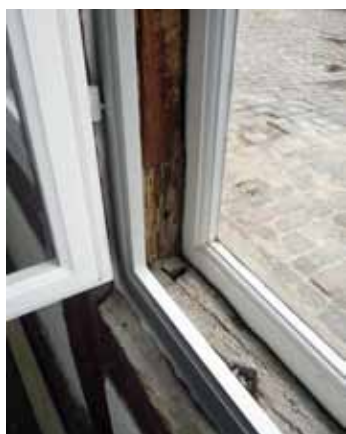
Faestnings Materialgard – Secondary glazing frames, Copenhagen, Denmark
