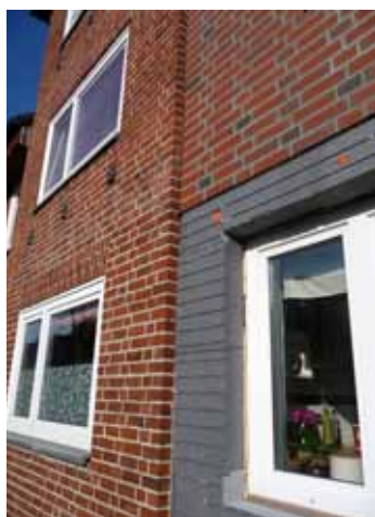
External wall insulation with brick tiles, Kiel, Germany
