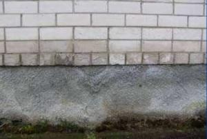
Internal thermal insulation is risky solution in cold climate: mould growth and condensation in the wall on the old wall surface
